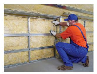
You also want to have the proper level of insulation in your crawlspace and in exterior and basement walls. The insulation under your floors only works when it is in contact with your house. If vou notice the floors insulation is falling, re-secure it with twine, wire, or lath.
